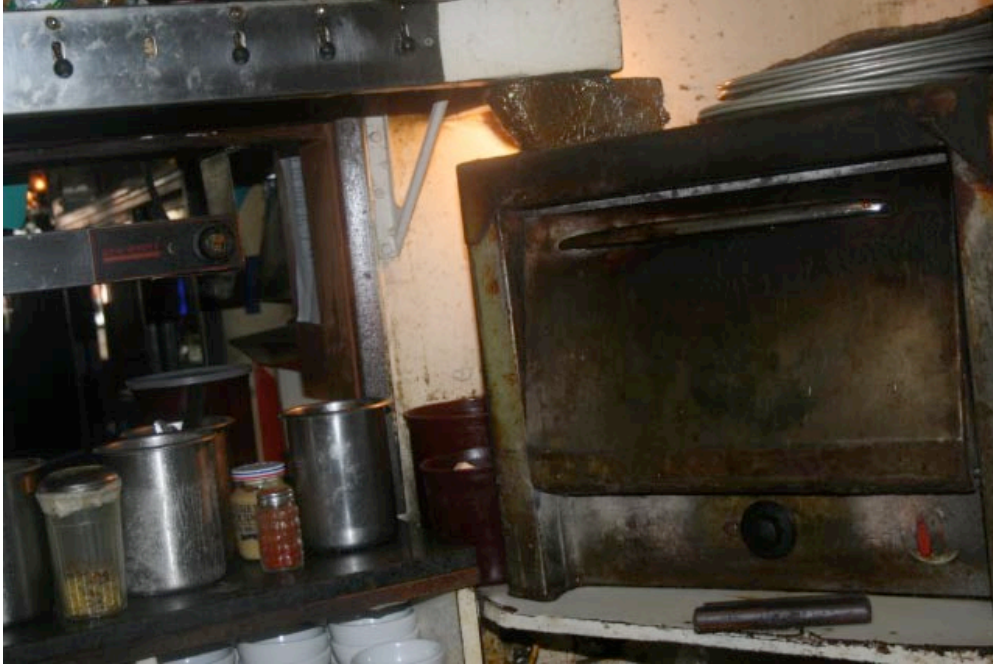
A fire at the popular East Bank Saloon damaged the kitchen and spread a greasy residue throughout the restaurant.
